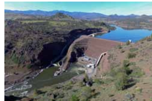
Iron Gate Dam. Photo: Mike Wier.
