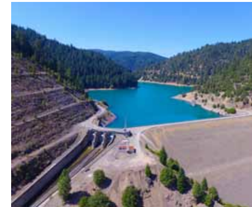
Construction of McCloud Dam in 1965 led to the demise of Bull trout in the McCloud River. Photo: Mike Wier.
