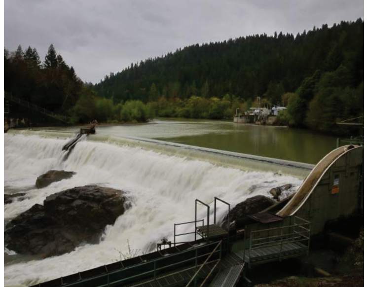
Water from the Eel River collects at Van Arsdale Reservoir and flows over Cape Horn Dam. A percentage of the water is redirected through a diversion tunnel to the Potter Valley Powerhouse and into the east fork of the Russian River. Photo by Christopher Chung / The Press Democrat
