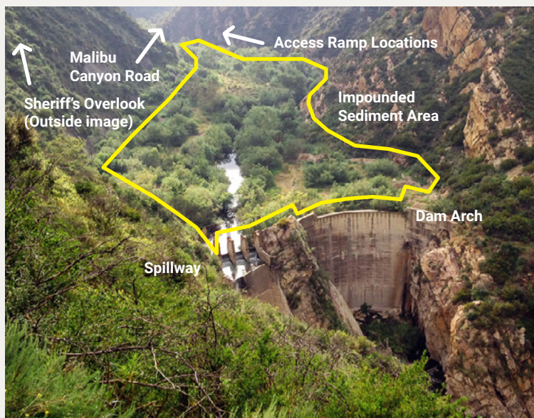
Rindge Dam structure, impounded sediment area and key reference points.
