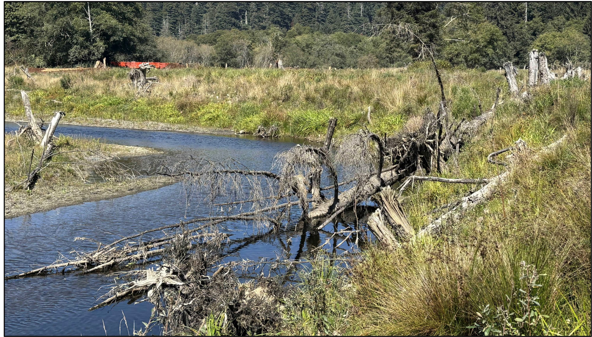
DETAIL 1: LWS INSTALLATION AND INTEGRATION ALONG STREAM BANK. PHOTO OF LWS INSTALLED AT PRAIRIE CREEK, HUMBOLDT COUNTY.
