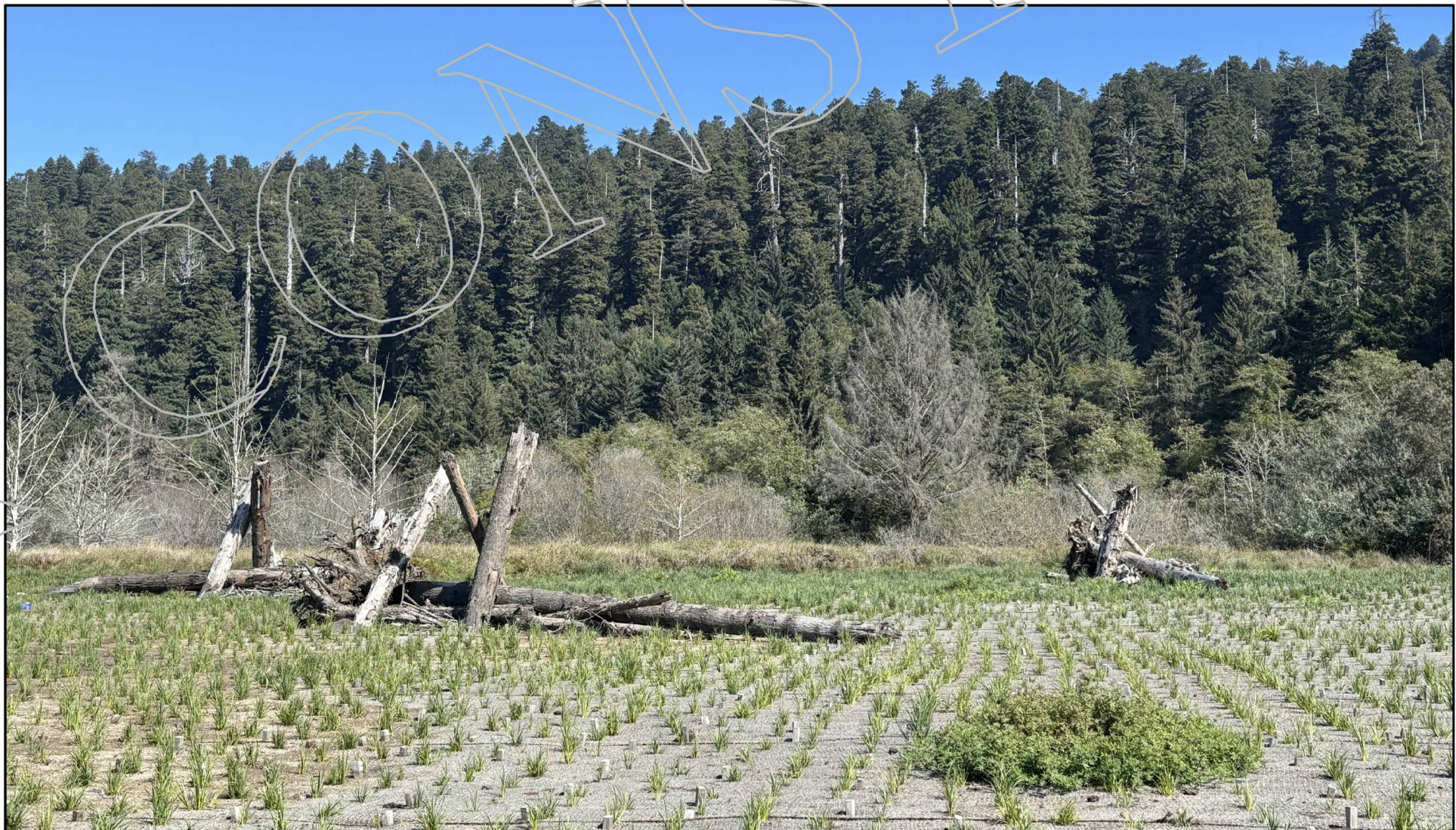
DETAIL 4: LWS INSTALLATION WITHIN FLOODPLAIN. PHOTO OF LWS INSTALLED AT PRAIRIE CREEK, HUMBOLDT COUNTY.
