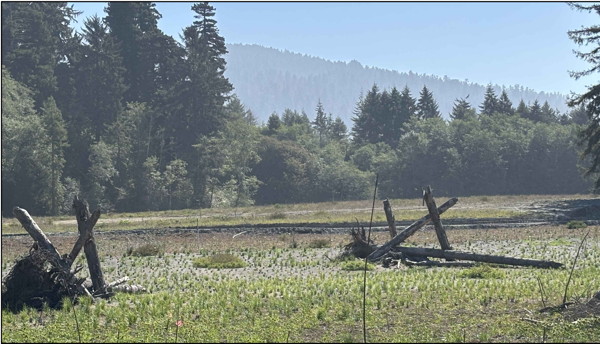
DETAIL 3: LWS INSTALLATION WITHIN FLOODPLAIN. PHOTO OF LWS INSTALLED AT PRAIRIE CREEK, HUMBOLDT COUNTY.
