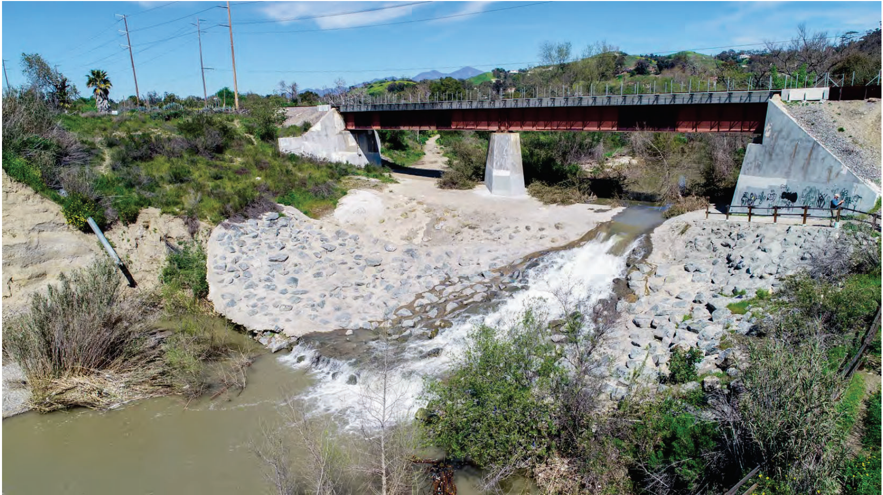
View to east - -looking upstream
